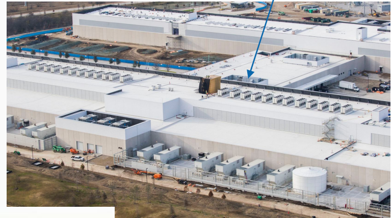
Meta datacenter in Texas
