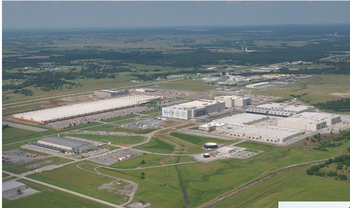
Google datacenter in Oklahoma
