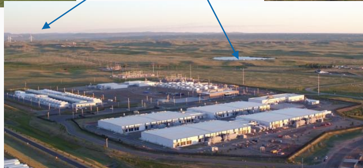
Microsoft datacenter in Wyoming
