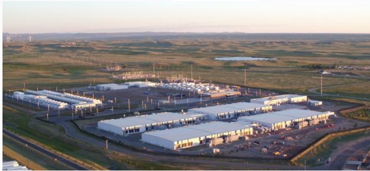
Microsoft datacenter in Wyoming
