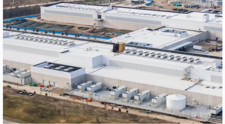
Meta datacenter in Texas
